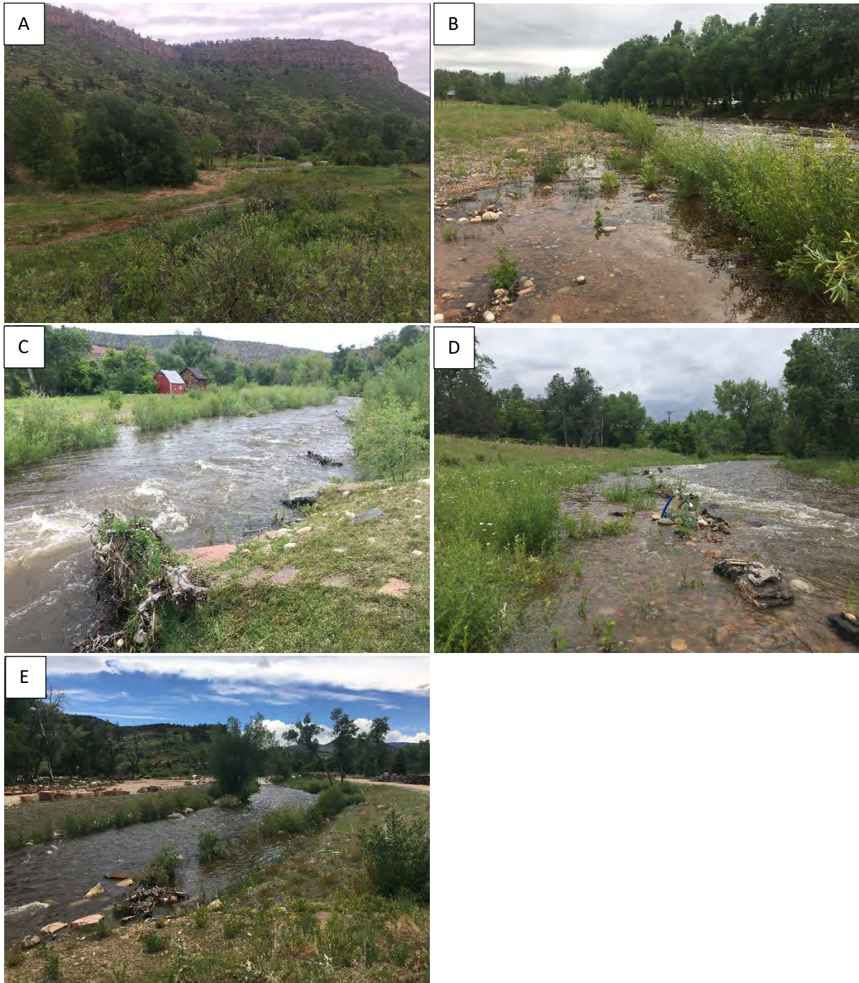
Figure 2. Annual peak flow observations from 6/21/2019 at restored sites in St. Vrain Watershed. Photo description match letter and arrow: A. activated side channel at Apple Valley North, North St. Vrain Creek; B. flows exceeding bankfull bench marked by willows at Apple Valley North, North St. Vrain Creek; C. flows exceeding bankfull bench marked by wood revetment and willows at downstream end of Apple Valley South, North St. Vrain Creek; D. flows exceeding bankfull bench marked by wood revetment at upstream end of Apple Valley South, North St. Vrain Creek; E. flows exceeding bankfull bench marked by willows at McConnell, St. Vrain Creek.
